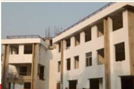
Ongoing Work – Macchodari School
